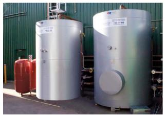
After commissioning, the system was powered on from 8am with a starting water temperature of 20°C. The system achieved 12,000 litres of storage at a temperature of 71°C by 3.30pm. Ambient temperatures were 10.9°C - 19.9°C.
